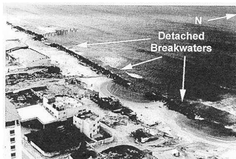
Fig 3: The detached breakwaters built in 1978 (Zviely and Klein., 2003)
