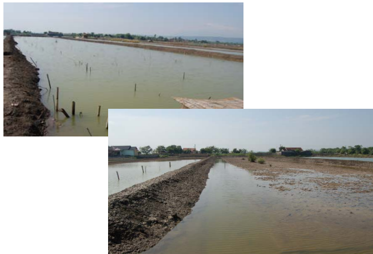
Shrimp pond condition before rehabilitation (left-above) and after rehabilitation (right-below)
