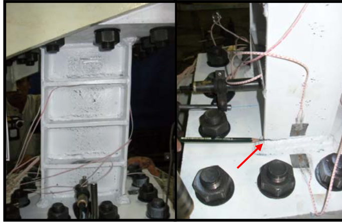
Figure 14 Fracture in the flange of the Specimen II at the top of the welded joints at the time of collapse.
