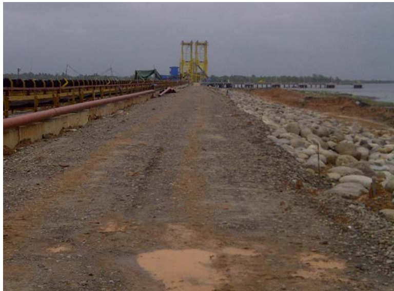
Figure 7 Causeway embankment after construction in Pangkalan Susu.
