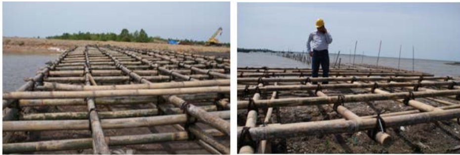
Figure 5 Gridded Matress Bamboo for Soft Soil Reinforcement.
