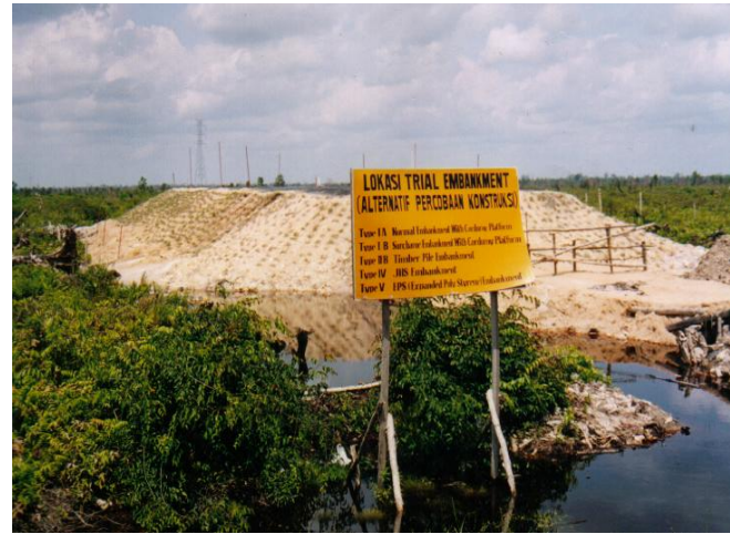
Figure 9 Trial Embankment Construction [1].
