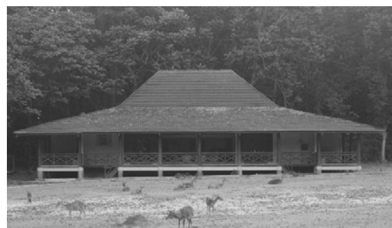
Figure 6. Resort building Flora A the large flat roof of which is one of the preferred PV locations
