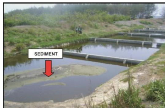
Figure 2. Zeolite tub at PT. IBD WWTP
