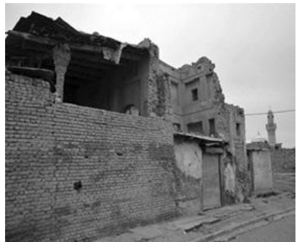
Figure 2: Deterioration of Citadel houses, Erbil
