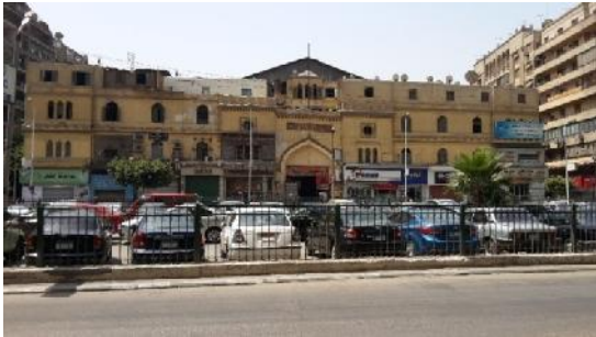
Figure 8. The marketplace in downtown, close to Tahrir square, has dwindled into a decaying state
