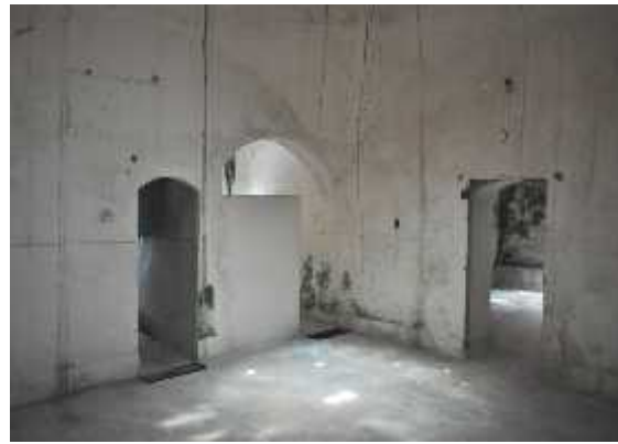
Figure 19. Hammam Al-Ward, Interior view of the Warm room
