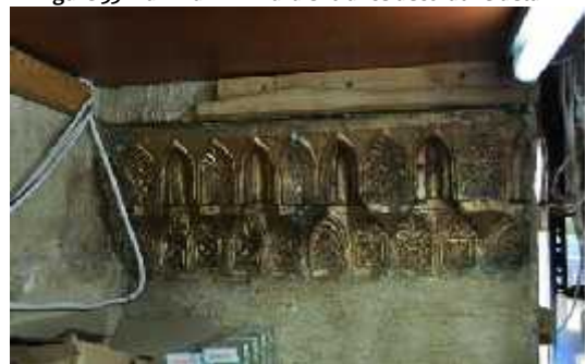
Figure 34. Hammam Al-Jadid entrance decorations
