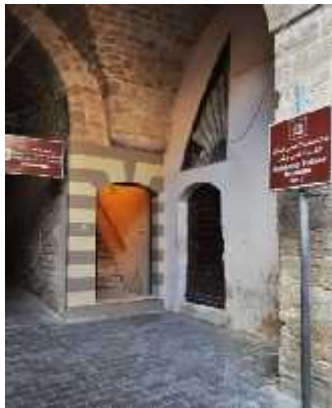
Figure 3. Khan al-Hummus/ al-Qishla (1721-1722) renovated between 2006 and 2010 by the Debbane Foundation
