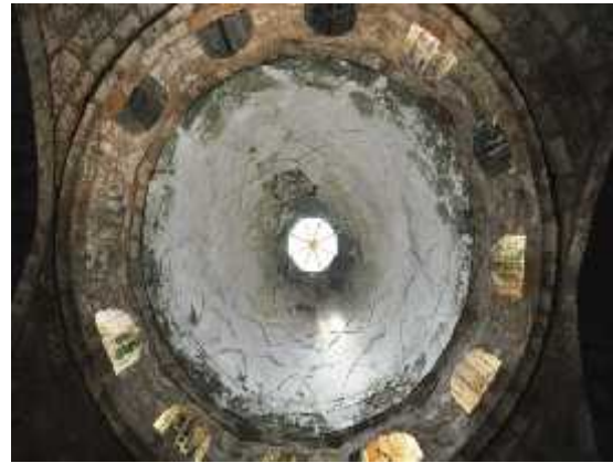
Figure 22. View of the dome over the Mashlah room
