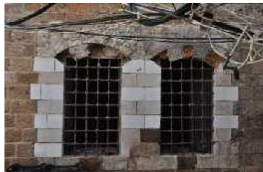
Figure 35. Hammam Al-Ward windows
