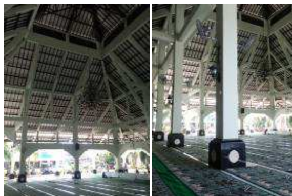
Figure 8. Body part of Sudirman Grand Mosque building (Source: survey, 2013)
