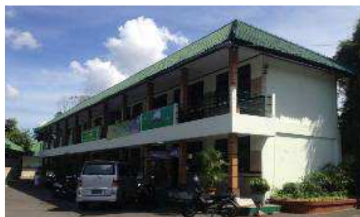
Figure 10. Supporting building of mosque (Source: survey, 2013)
