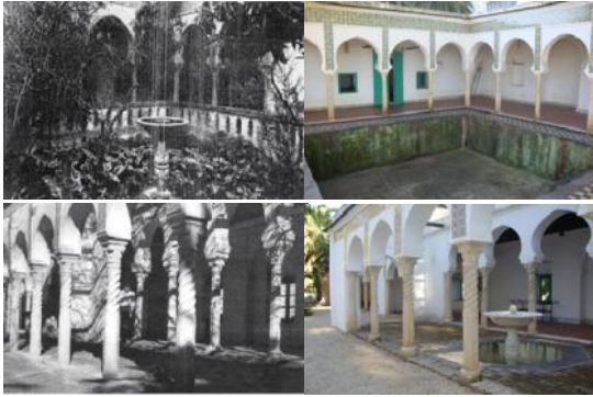
Figure 12. Architectural elements discovered during the restoration of the Djenane Abd-el-Tif (sources: IES archives of the Office National de Gestion et d'exploitation des Biens Culturels; Cazenave, E. La villa Abd-el-Tif : Un demi-siècle de vie artistique en Algérie 1907-1962, Association Abd-el-Tif, 2002, Paris, p. 26, 29; Photos: Personal collection, 2012)
