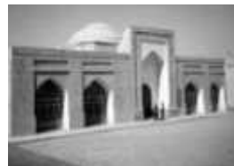
(c): Abdullokhon Mosque, 16 th century, Isfara, Tajikistan: the entrance [5]
