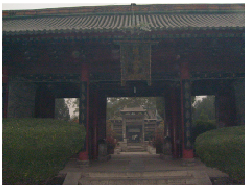
Figure 3. The influence of Chinese architectural style on Xi'an Great Mosque, China shown in the components of the mosque and its roofing
