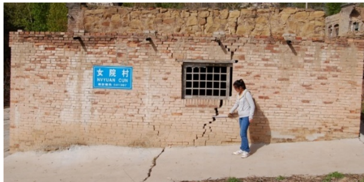
Figure 17 Case study of wall cracks.
