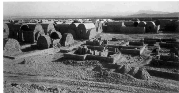
Figure 3. Maadher village under construction, the vaults for roofs. The work of Hassan Fathy has influenced this architecture
