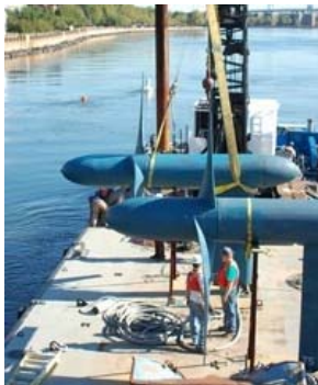
Figure 5. The turbines are transported to the RITE project site (Sep.2008) [14].
