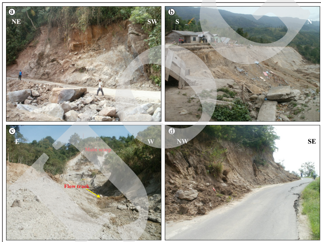
Figure 13. Photographs showing types of landslide triggered by the July 2, 2013 earthquake in a Gayo Highland area. (a) Rock fall of intrusive outcrop along the road to Kuta Panang, (b) A larger-scale landslide in Seurempah Village, (c) A dry earth flow triggered in the tuffaceous sand slope, (d) A surficial cut-slope failure along the roadside from Takengon to Blang Mancung.
