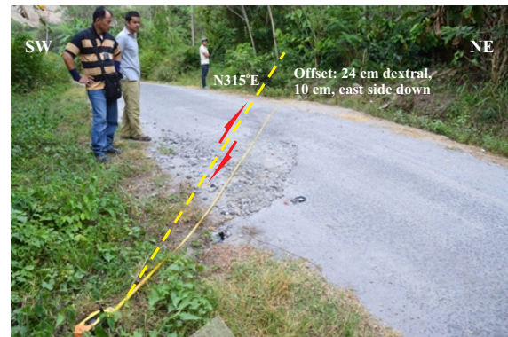
Figure 4. A photograph showing the surface rupture crossing the road between Kute Geulimai and Seurempah Villages. The rupture right-laterally displaced the road about 24 cm with a vertical displacement of about 20 cm, east side down.
