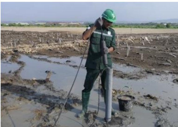
Gambar 52. Pemasangan open standpipe pm.
