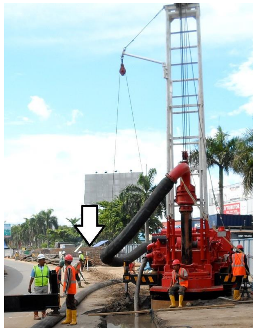
Gambar 3. Cek verticality alat bor (panah putih)
