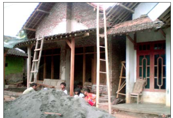
Figure 1. At the time of the study, there were people in every hamlet, especially the migrant workers' families, who were building new houses.
