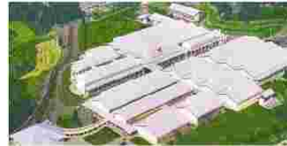
Figure 1.1. PT. Sido Muncul Plant at Ungaran-Central Java
