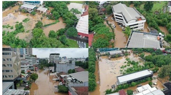
Figure 9. Flood-prone areas due to the overflow of the Krukut River
