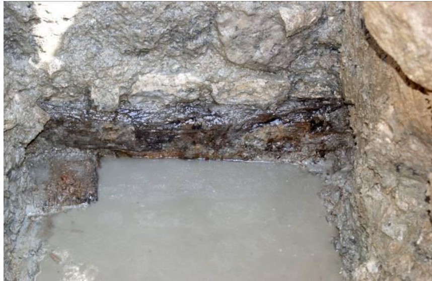
Fig. 3. Showing beam cross placed on to which the southern curtain wall rises, trench 2.
