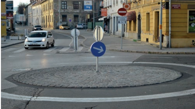
Fig. 6.17 Roundabout at a city intersection (mini-ring) [26]
