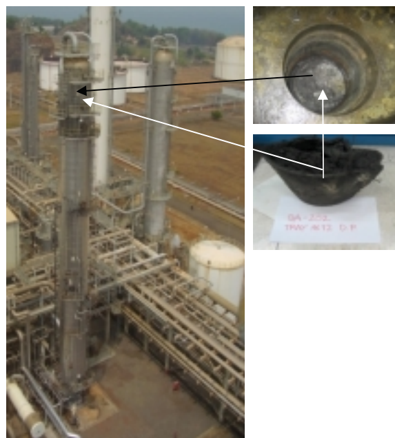
Fig. 9. Suspicious solidified material observed by gamma scanning was verified at the time of shutdown. A bucket buried in solidified mud was found on tray # 12 of DA-202 tower.
