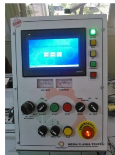
b. Unit Kontrol (main panel board)
