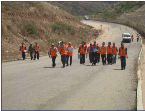
Participants in an IndII workshop inspect a new bypass in Bandung before it is opened to traffic. Courtesy of Phillip Jordan
