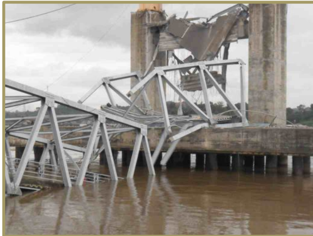
The collapse of the Kutai Kartanegara bridge in 2011, just ten years after it was constructed, highlighted problems with the rapid decay of existing infrastructure assets. Courtesy of Arief Rahman Saan (Ezagren)
