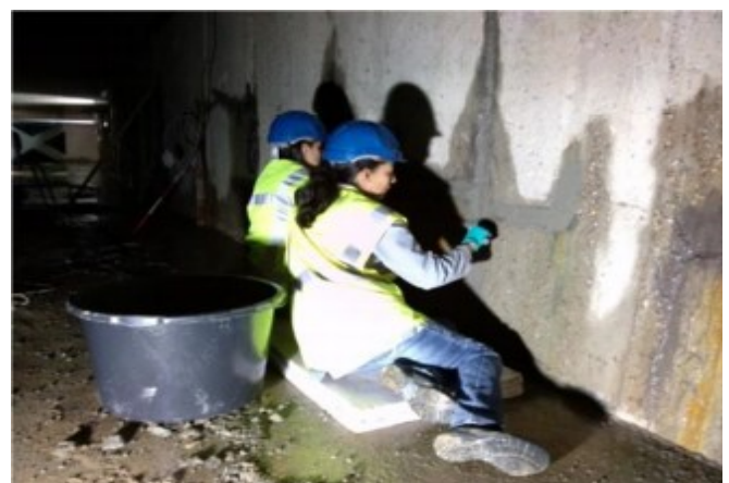
Figure 8. Application of bacteria-based self-healing repair mortar on actively leaking cracked concrete basement walls (Mors & Jonkers, 2019).
