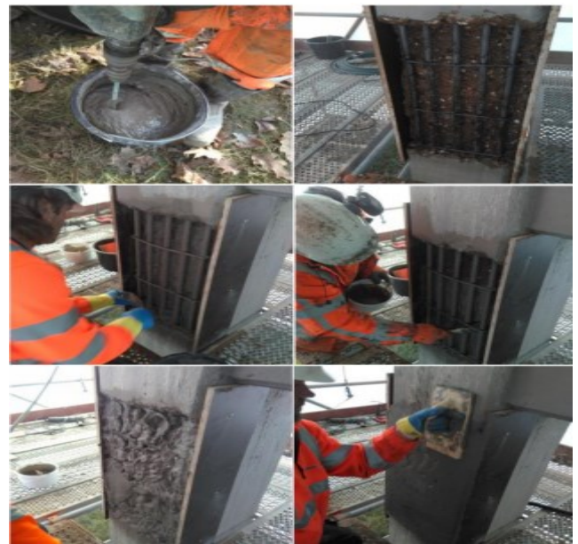
Figure 7. Application of bacteria-based self-healing repair mortar on steel reinforced concrete column (Mors & Jonkers, 2019).
