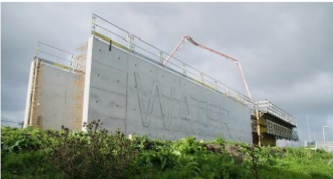
Figure 10. Full scale demonstrator in situ cast self-healing concrete water reservoir (Mors & Jonkers, 2019).
