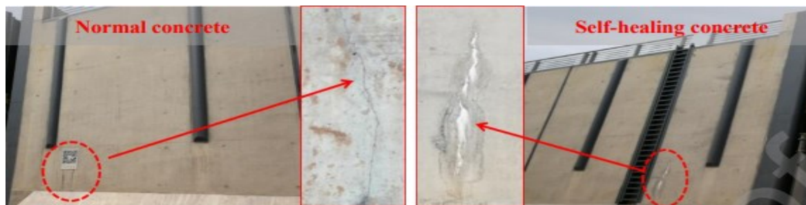
Figure 13. Comparison of self-healing effects of ship lock wall made by normal concrete (left) and made by bacterial concrete (right) (Zhang and Qian, 2020).
