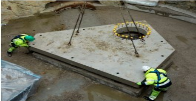
Figure 15. Roof slab made by bio-engineered concrete (Mulleem et al. , 2020).
