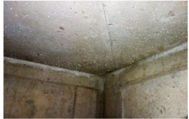
Figure 18. Condensation on the bottom side of the roof slab showing favorable condition for self-healing (Mulleem et al. , 2020).
