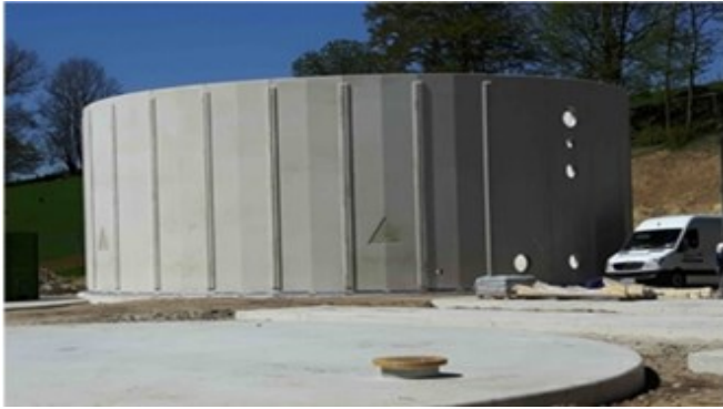
Figure 9. Prefabricated wastewater treatment tank by using self-healing concrete (under construction) (Mors & Jonkers, 2019).
