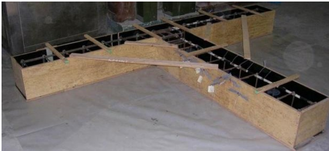
(a) Reinforcement and formworks
