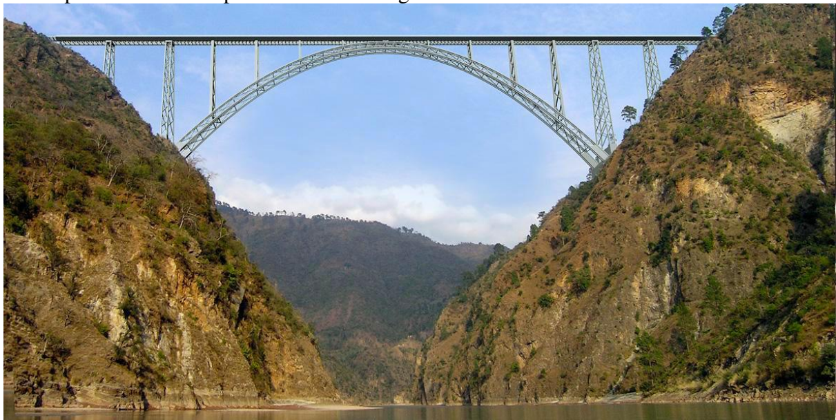
Figure 1: The Chenab bridge when completed
