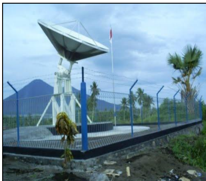
Gambar 4 Ground Station Bitung
