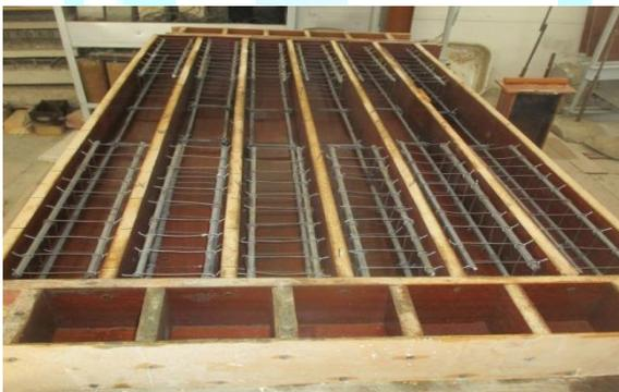
Fig.3. Crossbar formwork
