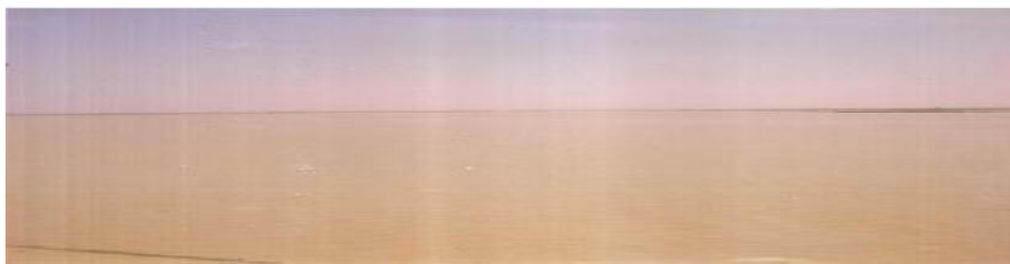
Plate 2. Different views of Jibia Dam which is used for irrigation in Jibia
