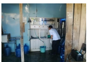
Figure 3. Floors that do not meet the requirements because there is stagnant water. Depot floors must be waterproof, flat, smooth, not slippery, not cracked, does not absorb dust, and is easy to clean, and the slope is sufficiently gentle to ease cleaning and no standing water.
