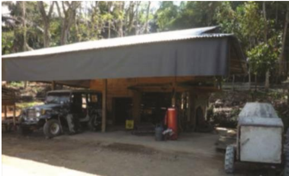
Figure 8. Turbine Manufacture Workshop owned by Multipurpose Community Group
