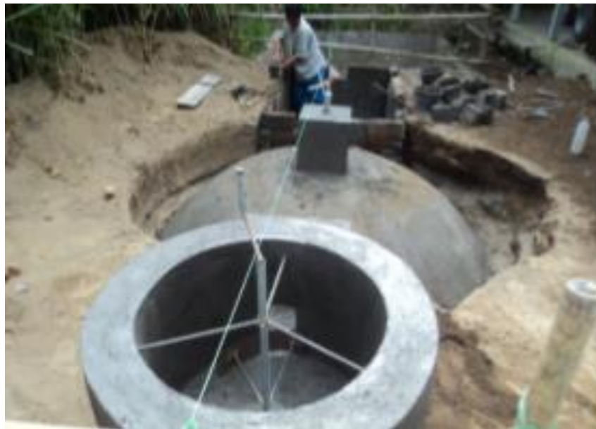
Figure 9. Biogas Construction with Community Participation
