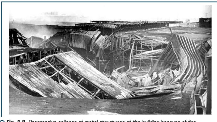
**Fig. 1.8** Progressive collapse of metal structures of the building because of fire
