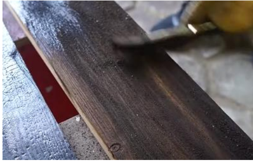
Figure 3. Surface Prep with Iron Brush [Source : Youtube Video [6]]
