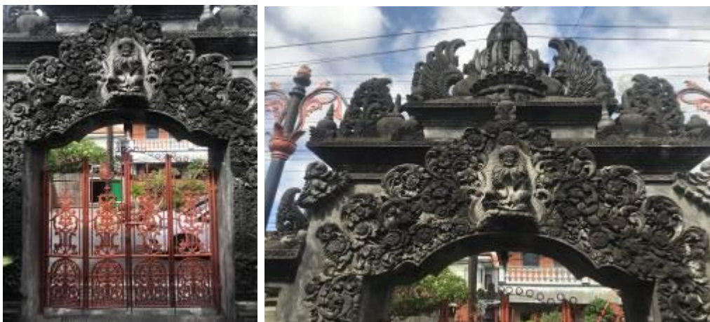
Figure 2. Al-Hikmah Mosque Entrance Detail [Source: Darmastuti, 2021]
