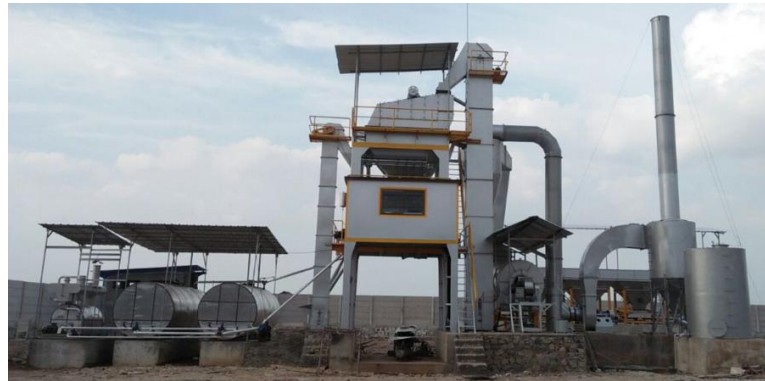
Gambar 1. Asphalt mixing plant
