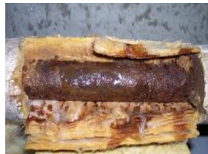
Gambar 2. Bocoran pipa akibat korosi
