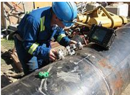
Gambar 4. PhasedArray Ultrasonic Test
