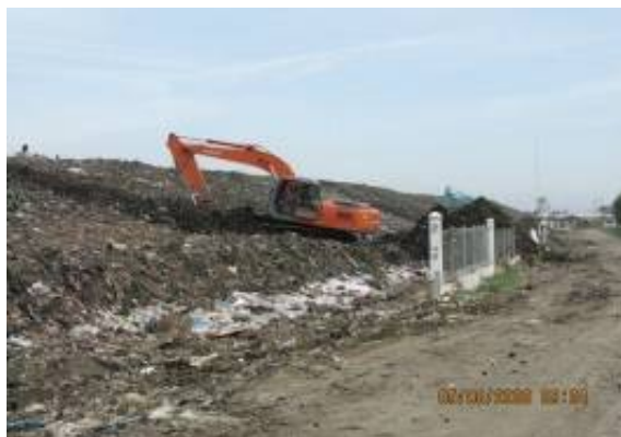
Figure 2. Rehabilitation of GJL in 2008
