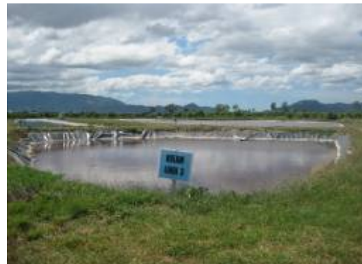
Figure 5. Leachate Treatment Ponds
