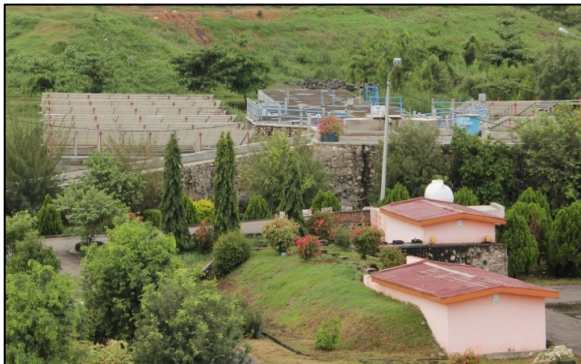
Figure 5. Closed WWTP utilizing DEWATS System, 85 m 3 Cap. (DK3, 2013)
