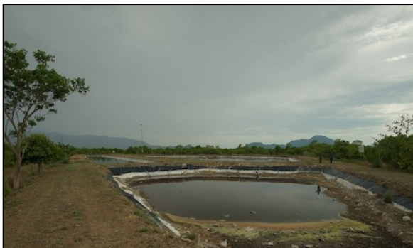
Figure 6. Pools for leachate treatment (Faisal, 2014)
