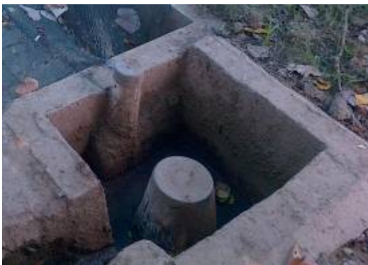
Fig 10. Inlet, cemented bricks
