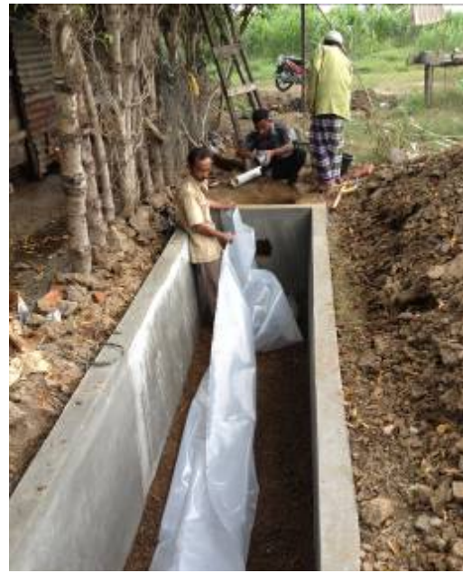
Fig. 9. Installation of plastic digester
