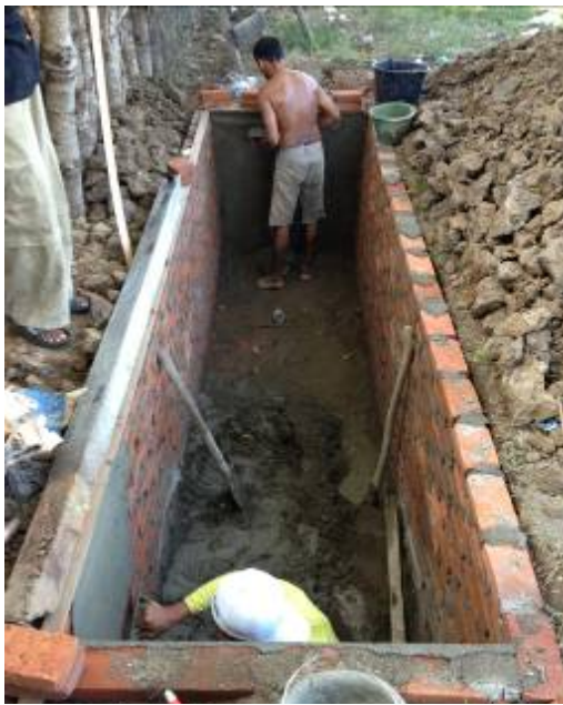
Fig. 8. Digester pit of plastered brick
