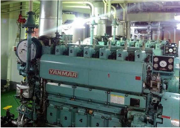
Gambar 2. Generator MV.SARI INDAH
