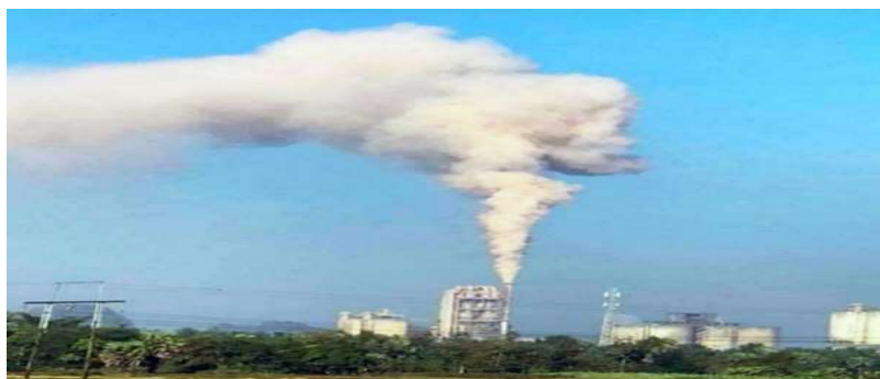
Figure 2: 4000 Tonne cement factory in Myaing Kalay, Hpa- an
