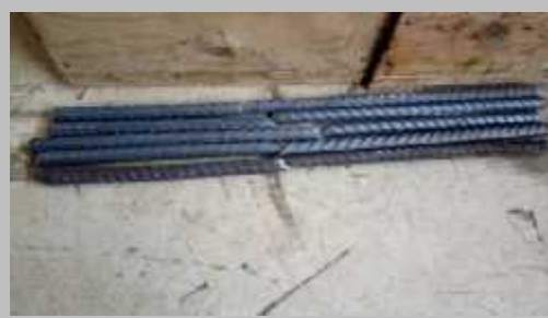
Figure 8. Photo of Reinforced bar
