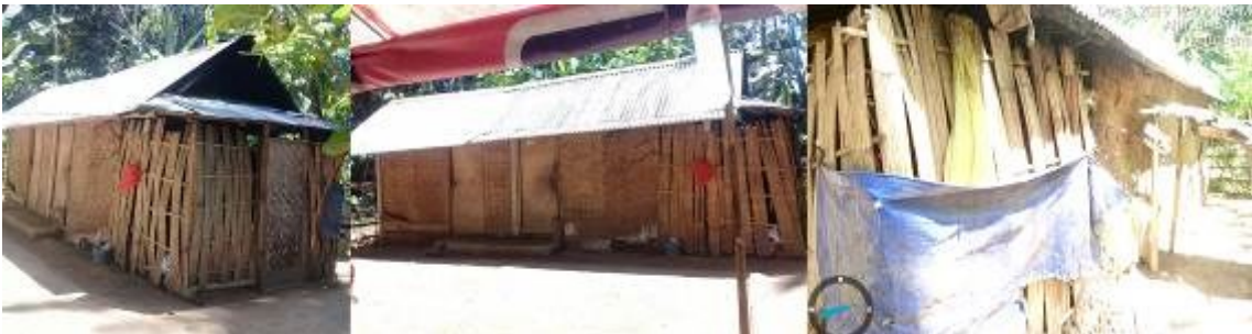
Figure 9: The condition of I Wayan Rena's house (one of the aid acceptor in Muncan Village)
