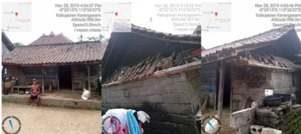
Figure 7: The condition of I Wayan Miada's house (one of the aid acceptor in Muncan Village)
