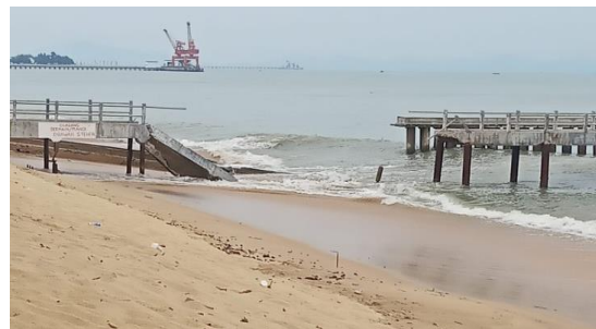
Fig 1. Damage of The Flying Bridge Due to The Impact of Pasir Panjang Beach Abrasion
