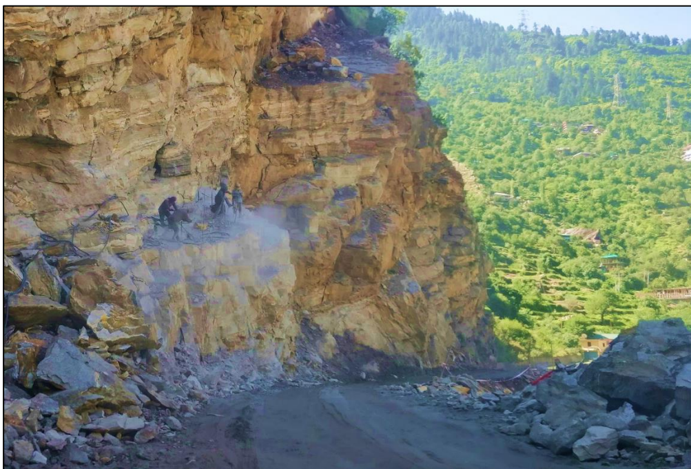
Figure 10. Road widening (Men at work) on NH-5 connect Shimla to Kaza via Kinnaur. Source: Primary Survey, 2017.
